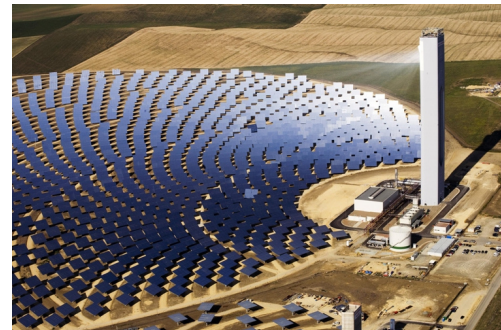
Solar tower power plant PS10, Spain.
